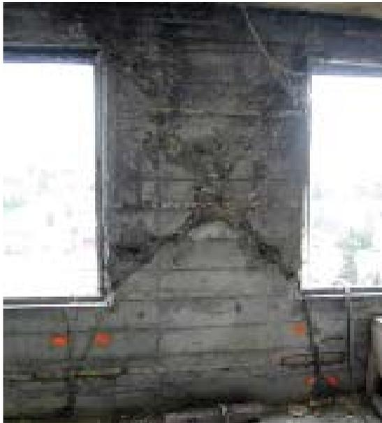
Fig. 1: Damage to walls caused by the earthquake
