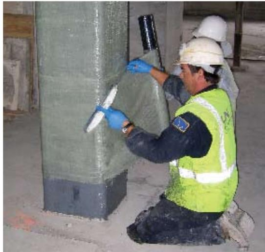
Fig. 3: Wrapping of columns with GFRP
