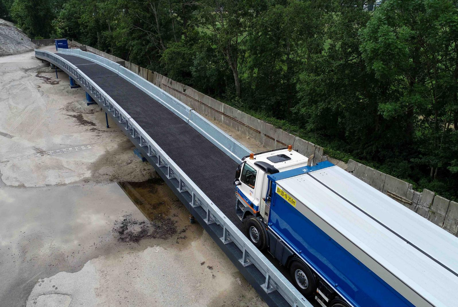
FiberCore's temporary composite bridge, HUGO, is placed 6.5 feet above the permanent structure and can carry all the bridge's normal traffic while repairs go on underneath.
