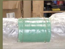
Apply epoxy to PipeMedic™ & wrap around packer ...
