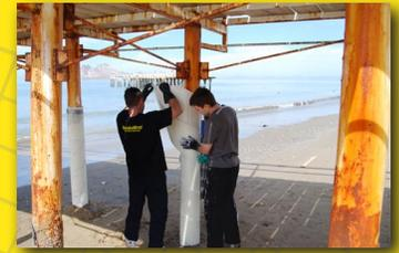
Apply epoxy to PileMedic™ and overlap to create a continuous seamless shell
