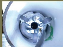
Guide to repair position w/ CCTV camera; inflate packer...
