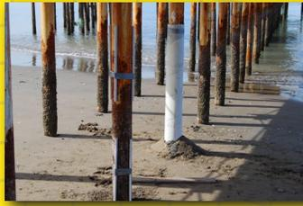
Attach spacers to damaged Pile
