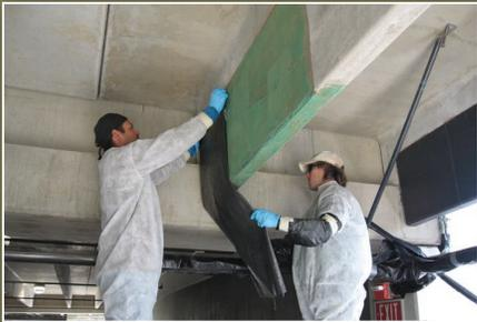
Introduced in the 1980s by QuakeWrap President, Professor Mo Ehsani, Carbon Fiber Reinforced Polymer (CFRP) is a structural reinforcing material that is applied like wallpaper, reaching 2 to 3 times the strength of steel in 24 hours.
