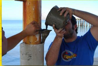
Allow underwater epoxy to cure. Inject grout or resin & remove spacers
