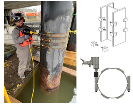
Fig. 4. ShearClamp™ used on H-piles and ShearWrap™ steel bands that are torqued around circular steel piles.
