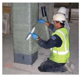
Fig. 3: Wrapping of columns with GFRP
