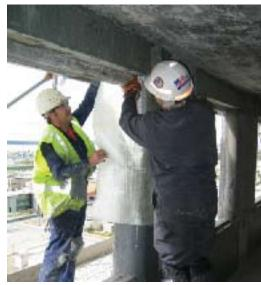
Fig. 5: Reinforcing boundary elements in shearwalls with GFRP
