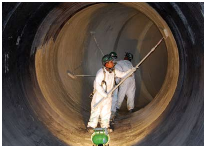
Application of final finish coating over installed FRP
