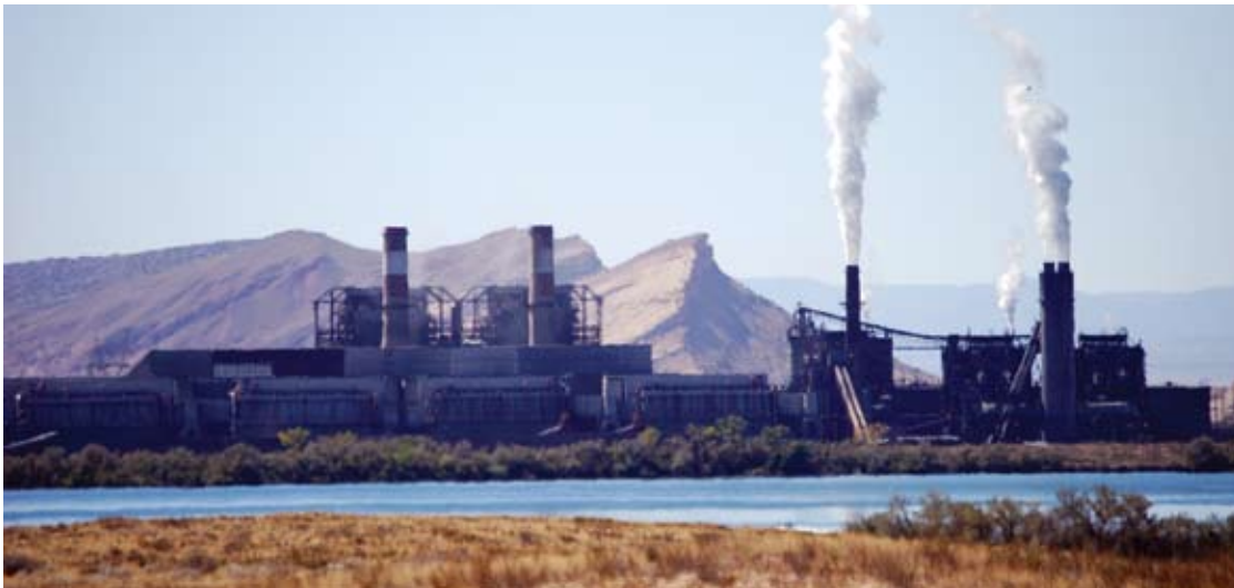
San Juan Generating Station, New Mexico
