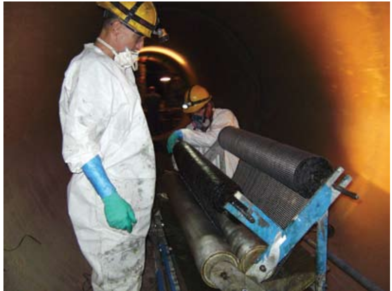
Saturating machine reassembled inside the pipe
