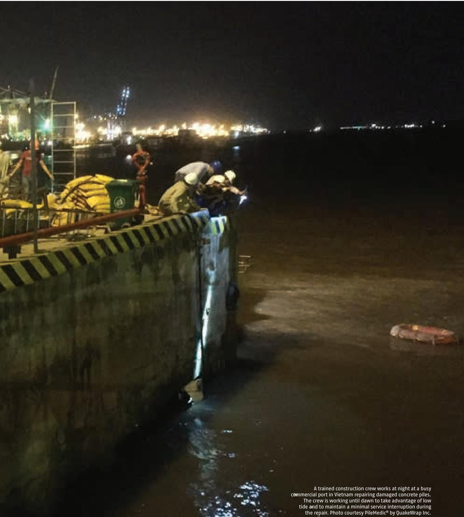
A trained construction crew works at night at a busy commercial port in Vietnam repairing damaged concrete piles. The crew is working until dawn to take advantage of low tide and to maintain a minimal service interruption during the repair. Photo courtesy PileMedic® by QuakeWrap Inc.
