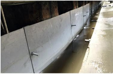
The Sheet Pile Repair (SPiRe®)system is an innovative new system of **repairing and restoring corroded steel sheet piles**, both above and below water, using FRP composites\*
