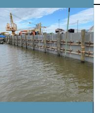
The SPiRe® by QuakeWrap repair system significantly reduces corrosion by inhibiting both oxygen and water from reaching the structure. Here are the advantages and benefits that make SPiRe® stand out for repair of inland commercial infrastructure:
