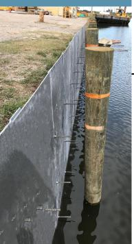
The Sheet Pile Repair or SPiRe® system made exclusively by QuakeWrap is constructed with **lightweight** honeycomb or 3D fabric sandwiched between sheets of **resin saturated FRP** fabric. These panels may be custom prefabricated to match the shape of the steel bulkhead or concrete seawall being repaired.
