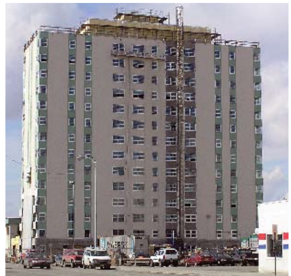
Fig. 6: The building nearly completed and painted
