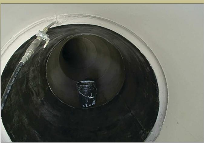
Figure 2. A post-installation picture from the first application of StifPipe<sup>®</sup> by sliplining. Note the grout injection port used to fill the annular space.
