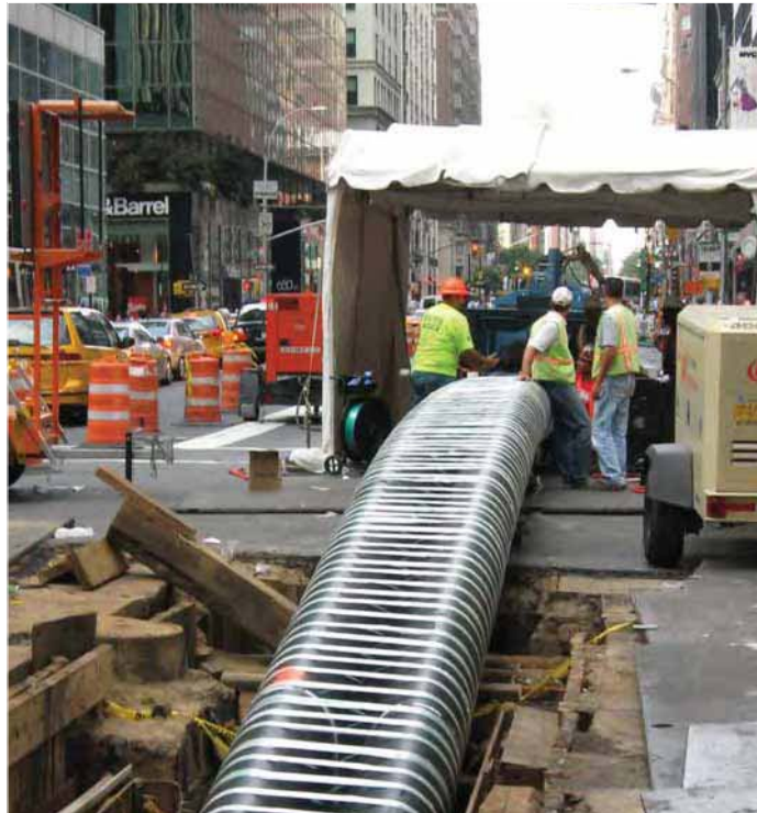
To date, more than 5,200 ft of water main has been renewed.
