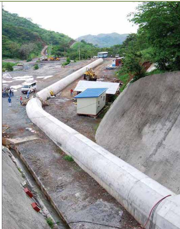
The repair involved using a fiber-reinforced polymer.
