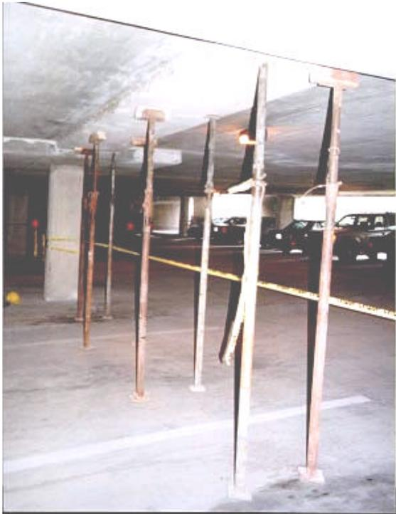
**Figure B.2: Shoring on floor above tested slab**
