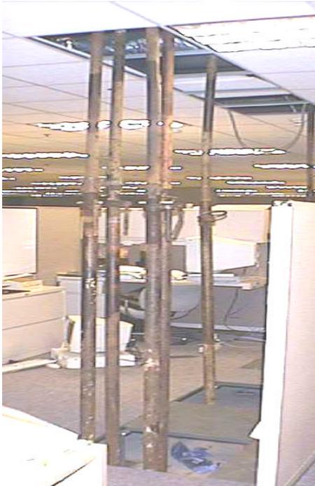
**Figure B.4: Shoring in place for push-down method**
