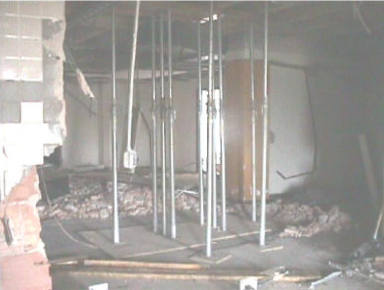
**Figure A.9: Typical shoring setup on the floor above the test member**
