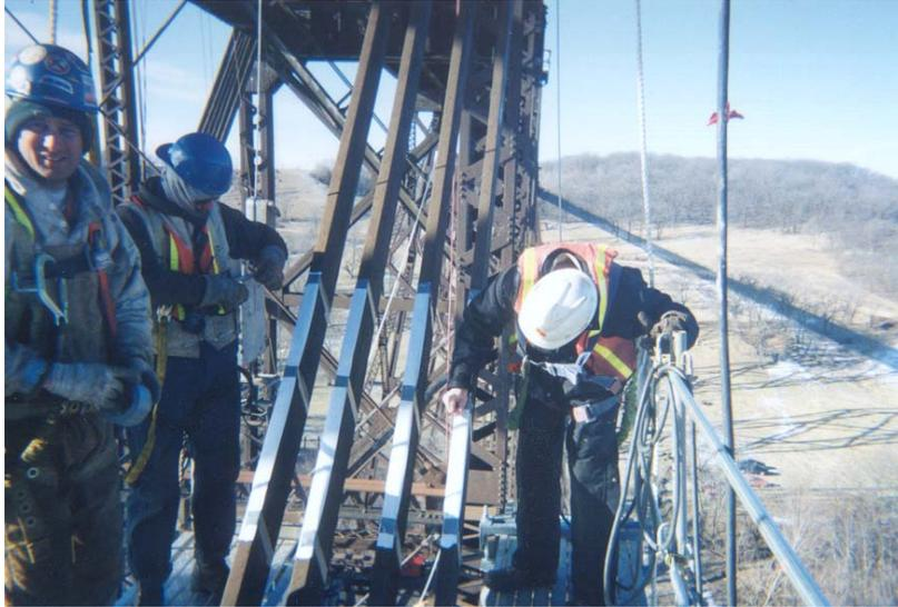
**Figure 8-13 Manually Investigating the Tightness of Eyebars in Steel Bridges**
