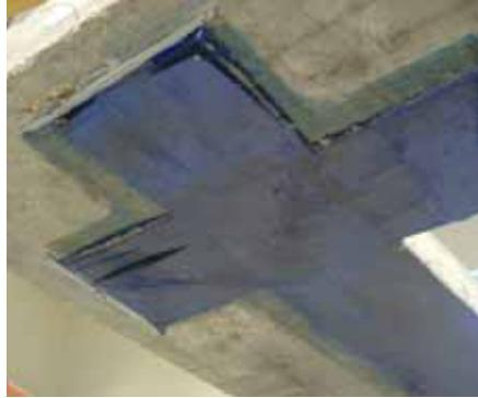
e) Delamination of the CFRP plies on one corner
