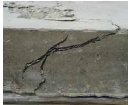
b) Shear crack along the support side
