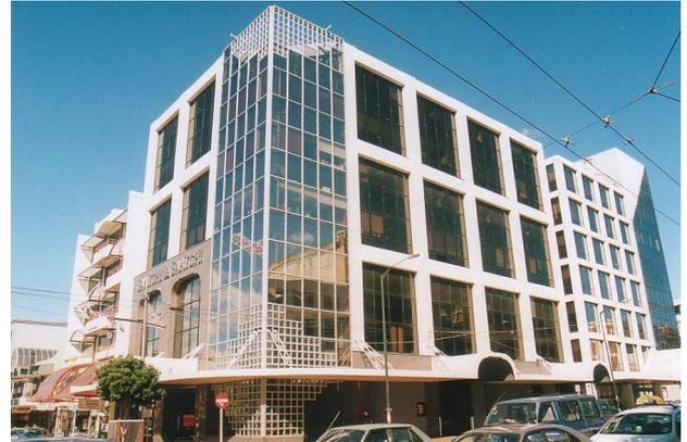
Saatchi & Saatchi House was constructed in the late 1980's. There was a tolerance problem with the construction of the columns, which was corrected with a thick plaster. This plaster was applied in several layers and to varying thickness of up to 70mm. Generally recognised good trade practice was not followed in the application of the plaster, and there were many areas where the plaster had cracked and delaminated from the concrete substrate or within the inner layers of plaster.
