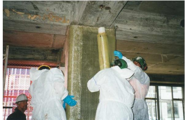
In 1999, a twelve-storey office building in Wellington CBD was converted into the IBIS Hotel. Contractor Fletcher Construction engaged Contech to carry out seismic strengthening of the structure using FRP Composite Material. Structural analyses carried out by Holmes Consulting Group indicated that sixteen columns on the first four floors of the building did not meet the NZ Code requirements.
