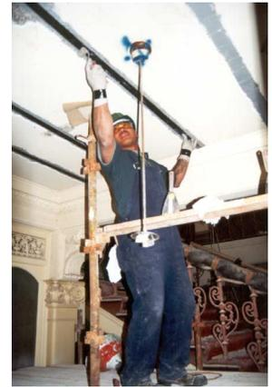
Structural strengthening has been used for many years to extend the service life of important and historical buildings and structures around the world. Traditionally, this type of retrofitting has utilised bonded steel plates or external post-tensioning. However, with the advent of composite materials consisting of synthetic fibres of E-glass, Kevlar and Carbon, immersed in a matrix of epoxy resin, the means of strengthening these structures has been significantly simplified.
