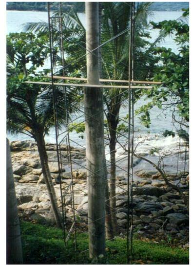
The luxurious Amanpuri Villas, on the island of Phuket, Thailand, are built on slender concrete columns of 300mm diameter, up to 14.0m high. With the ocean located only 30m from these villas, the columns have been subjected to the forces of the environment, since their construction 10 years ago. Most of the columns exhibit corroded rebar and spalled concrete.
