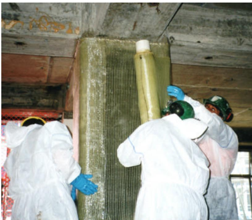
*Fig 5.2: Application of saturated BBR GFS to column*
