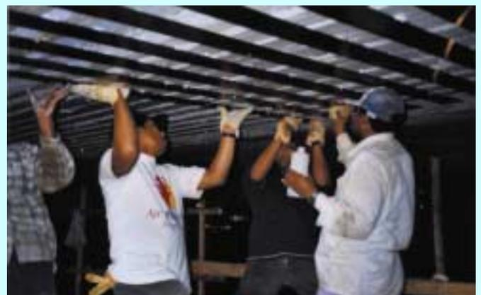
*Application of CFRP laminates to bridge deck*
