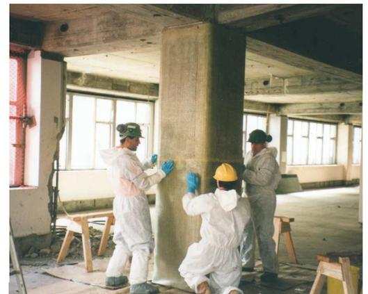
Over 450m<sup>2</sup> of FRP composite material and more than 400 fibre anchors were installed on this project. The crew of 4-6 men completed the whole work, including column preparation, over the stipulated period of four weeks.
