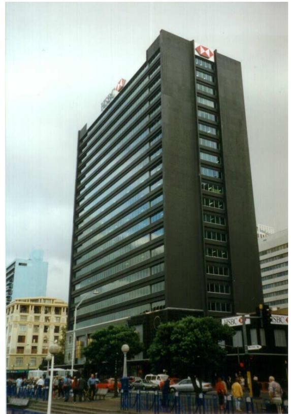
The HSBC Building, formerly the Air New Zealand Building, was built in the late 1960's and in 1998 underwent a complete internal and external refit. Externally, the podium was clad in black marble and the tower block, which consisted of in-situ columns with a textured plaster finish and precast spandrels, was painted a dark green. The plaster on the columns, generally up to 40mm thick began to delaminate and sections fell to the footpaths below.
