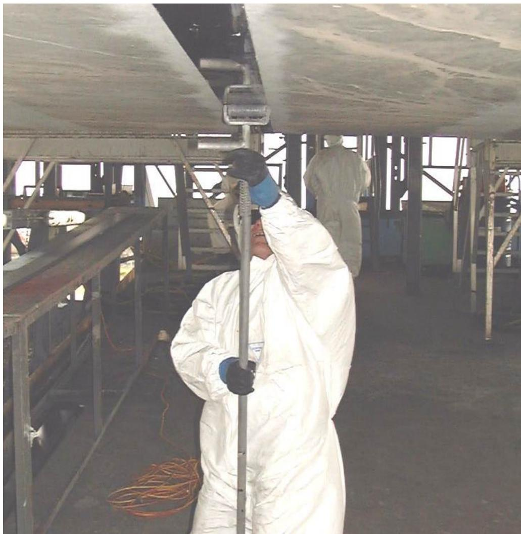
*Fig 5.3: Application of the CFRP laminate*
