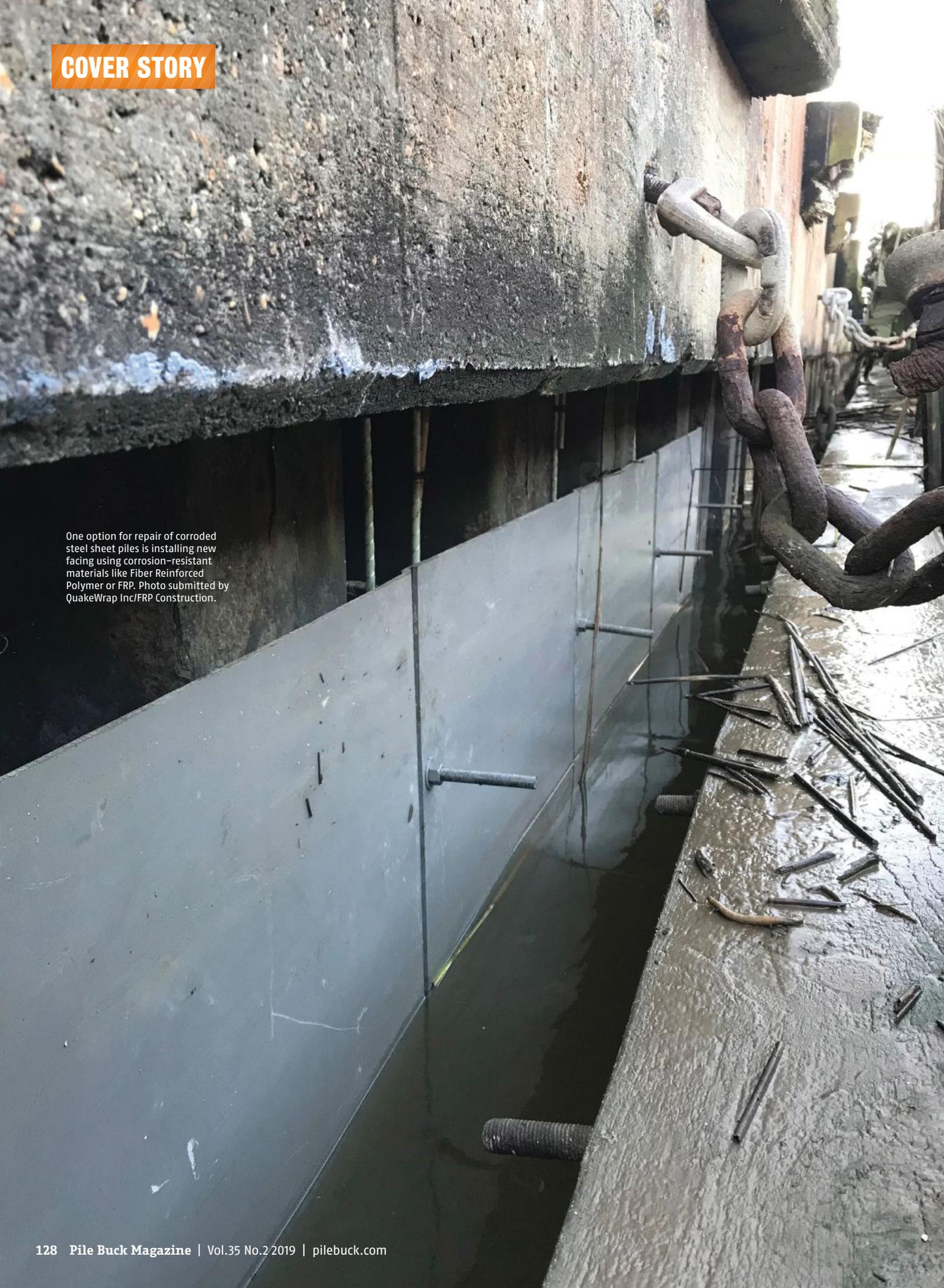
Again, the material used must be resistant to the erosive action of the waves and corrosive action of the seawater. The material used to fill in the annular space between the new FRP facing and the deteriorating bulkhead wall needs to be an inert
