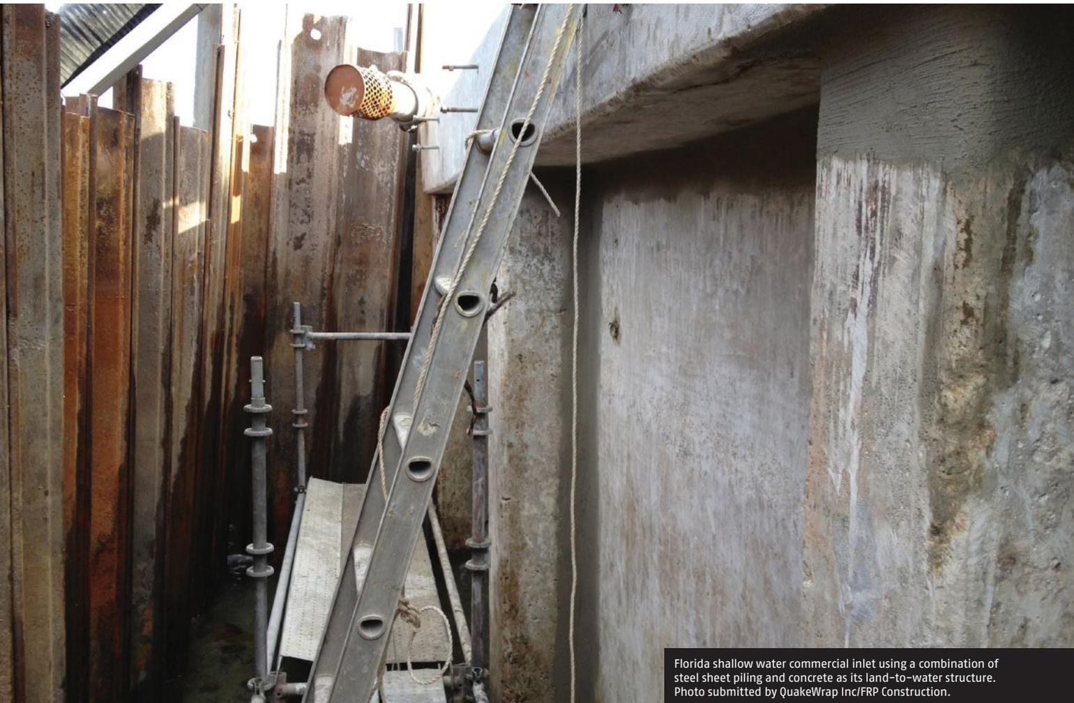
Florida shallow water commercial inlet using a combination of steel sheet piling and concrete as its land-to-water structure. Photo submitted by QuakeWrap Inc/FRP Construction.
