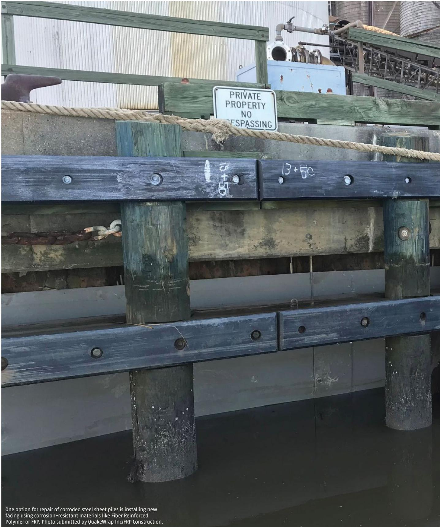
One option for repair of corroded steel sheet piles is installing new facing using corrosion-resistant materials like Fiber Reinforced Polymer or FRP. Photo submitted by QuakeWrap Inc/FRP Construction.
