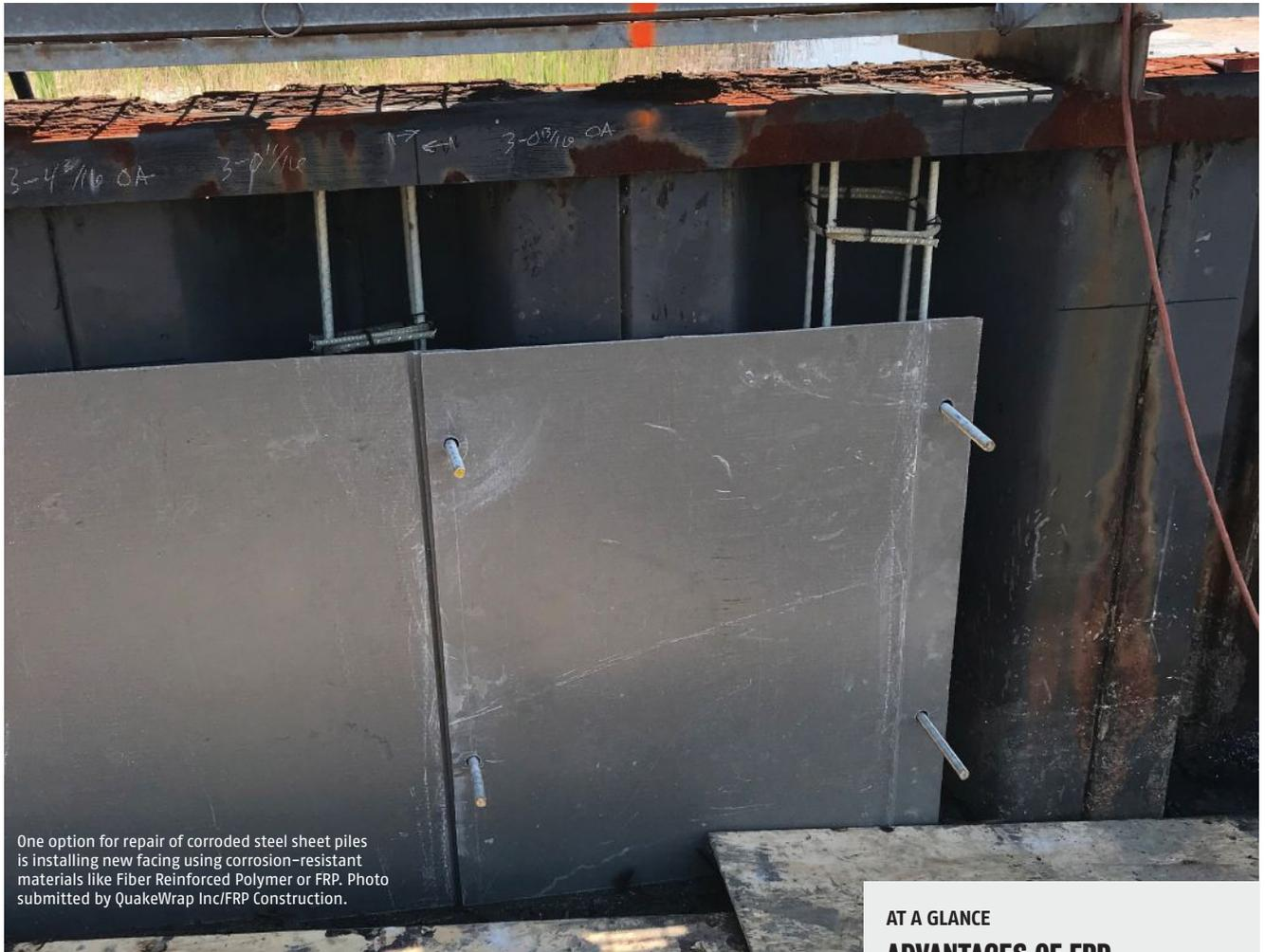
One option for repair of corroded steel sheet piles is installing new facing using corrosion-resistant materials like Fiber Reinforced Polymer or FRP. Photo submitted by QuakeWrap Inc/FRP Construction.
