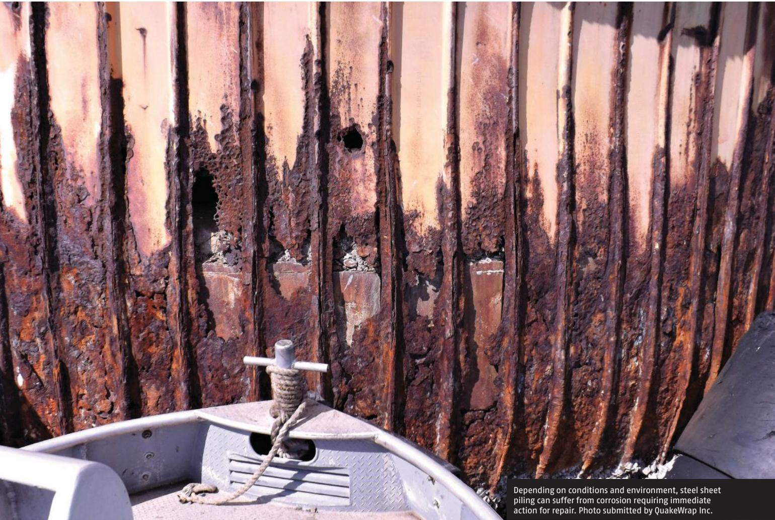
Depending on conditions and environment, steel sheet piling can suffer from corrosion requiring immediate action for repair. Photo submitted by QuakeWrap Inc.
