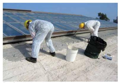
Fig. 4: Smoothing the rough concrete deck
