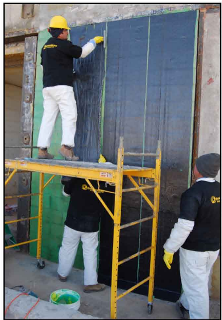
Figure 1: CFRP fabric installation on URM wall
