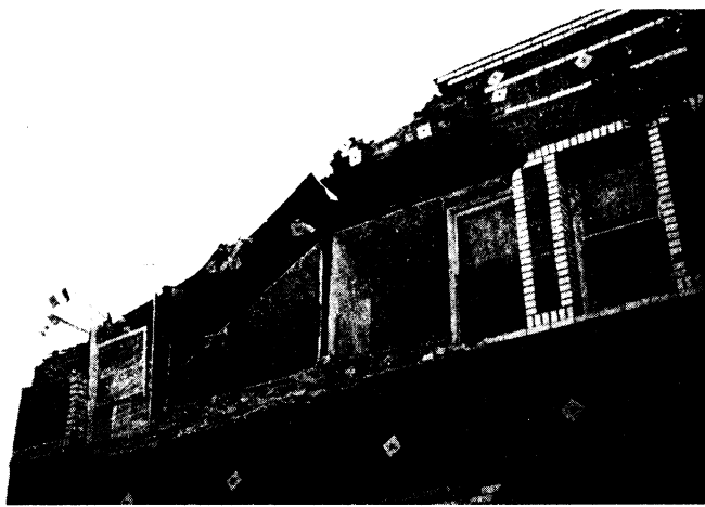
FIG. 2. Failure of URM Wall That Was Retrofitted by Tying Floor Beams to Wall
