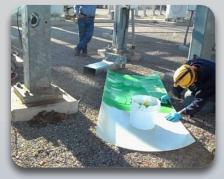
Cut a piece of PileMedic<sup>™</sup>, apply epoxy & wrap ...
