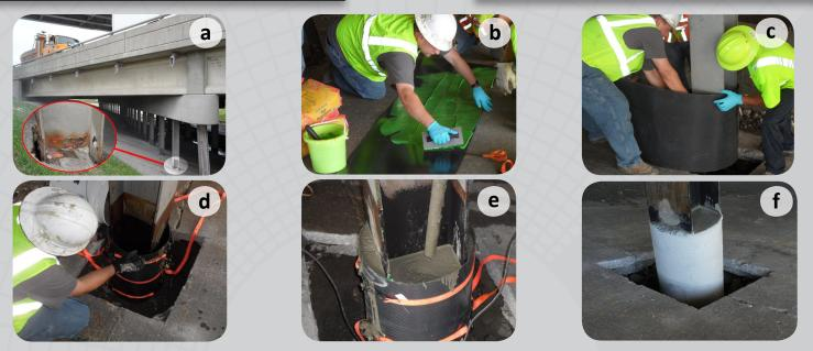
a. Corrosion-damage b. Apply epoxy to PileMedic<sup>\*\*</sup> c. Wrap PileMedic<sup>\*\*</sup> around column or pile to create a cylindrical shell d. Temporarily support shell w/ ratchet straps e. Fill annular space with grout f. Remove ratchet straps & paint jacket (if desired)
