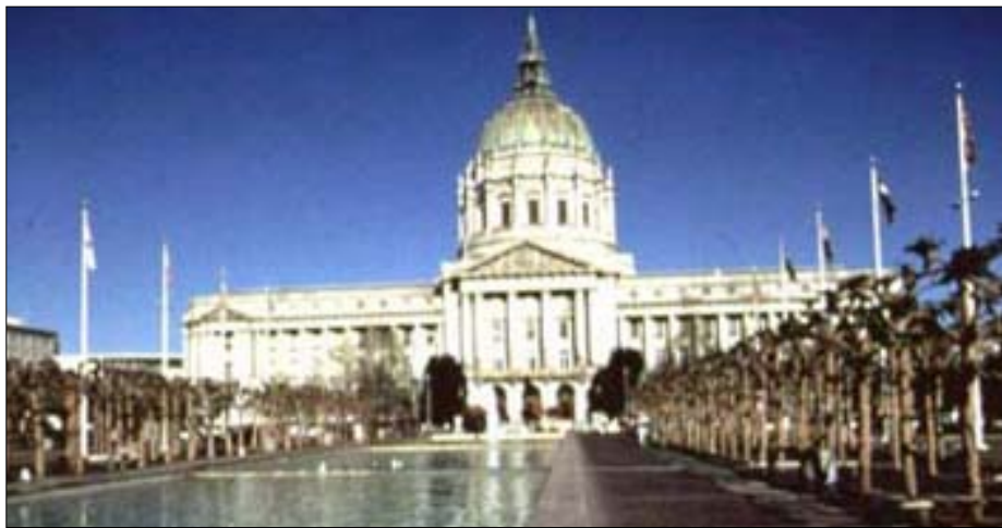
San Francisco City Hall Retrofitted hollow clay tile walls in basement
