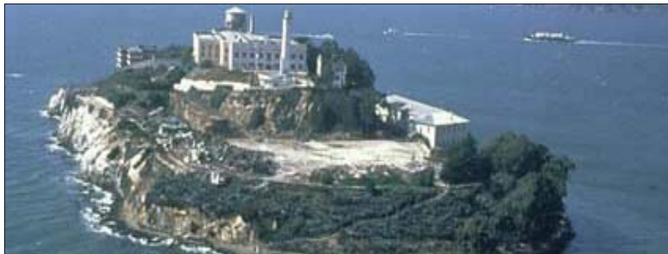
Alcatraz National Park, San Francisco, CA Retrofitted masonry smoke stack
